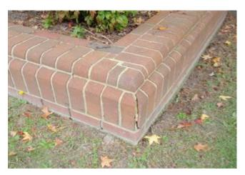
While they may need periodic cleaning these expenses are considered maintenance items. The walls display a small amount of damage believed to be reckless groundskeeping. Some mortar joint erosion is beginning to appear in areas. These conditions were noted in the previous study (2019) and no work appears to have been performed.
